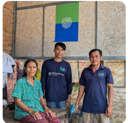
Repairing Chan Toch's house
